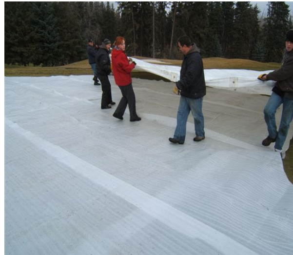
Figure 4. Tarps placed over vent tubes.
